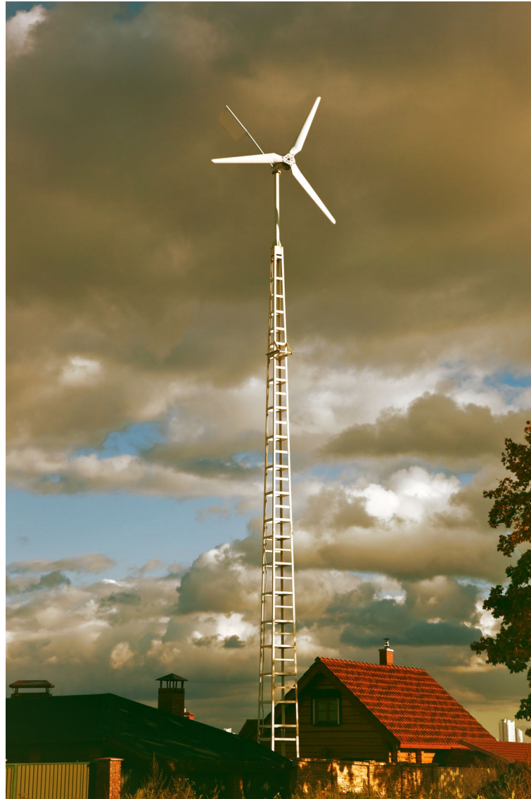
Figure 34. Small wind turbine for domestic use.
